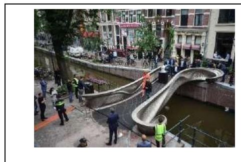
MX3D Bridge: fully functional stainless-steel bridge [2]
