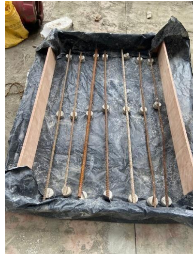
Figure 8: Laying of different types of rebar
