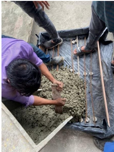
Figure 9: Concreting of the mould
