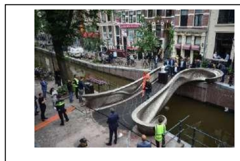
MX3D Bridge: fully functional stainless-steel bridge [2]
