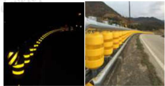
Fig.5 Rolling Barriers during Night and Day Time
