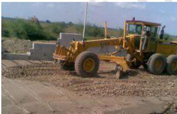
Grading of Fill Material
