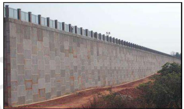
Building Sector (Boundary walls)
