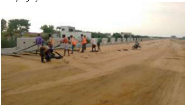
Laying of ParaWeb
