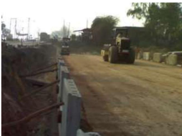
Rolling and compaction of soil
