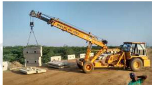
Erection of Panels
