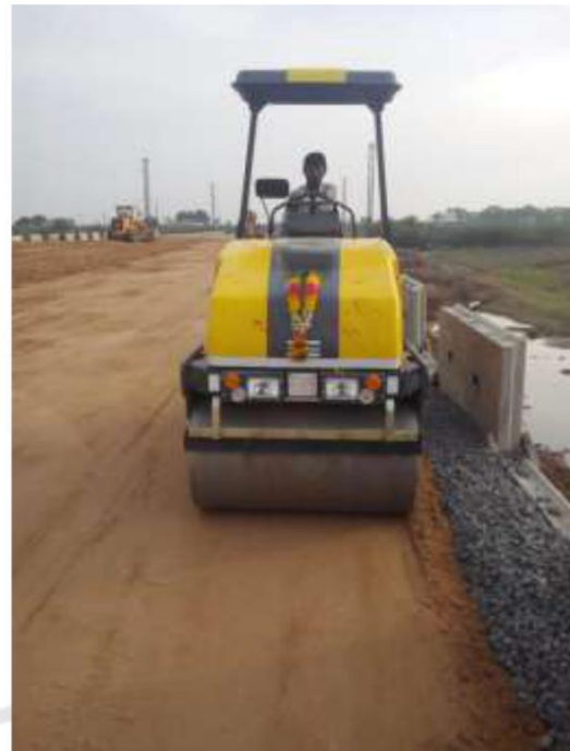
Compaction with 1 ton roller immediately behind the panels.
