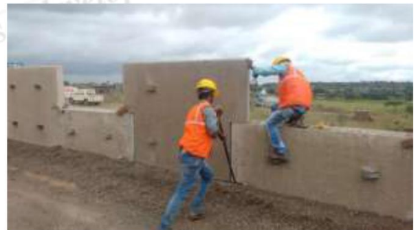
Alignment of Panels
