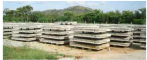
Stacking of Panels
