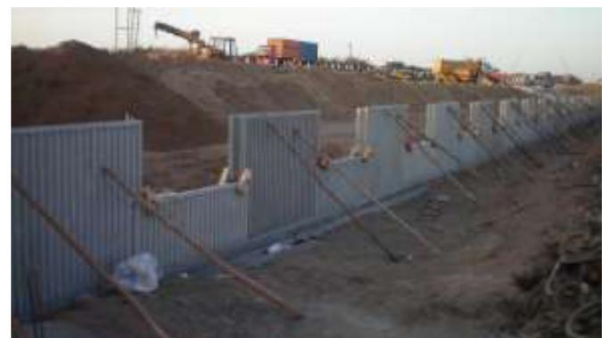
Timber supports to prevent over-turning
