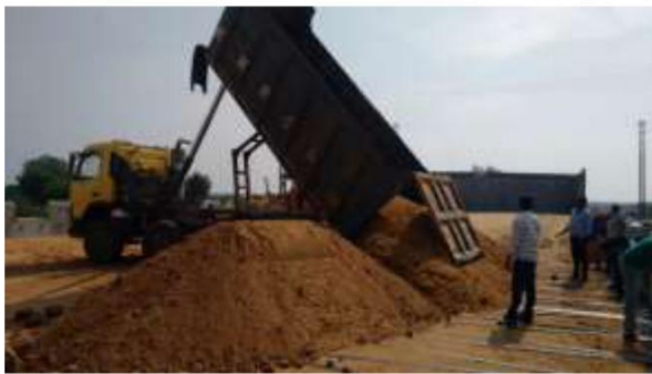
Dumping of Fill Material
