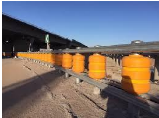
FIG NO.03 COLLISION RESISTANT ROLLERS
