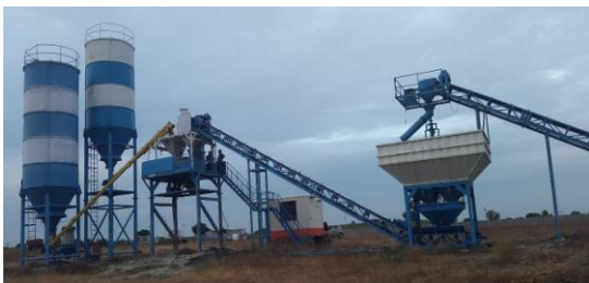
Fig no.1.1 Layout of RMC plant
