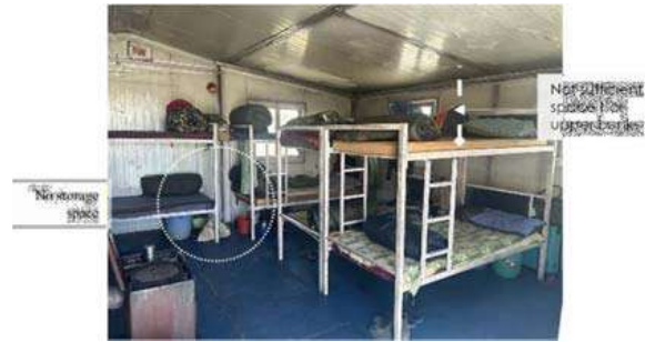
Figure 9: Interior of Shelters
