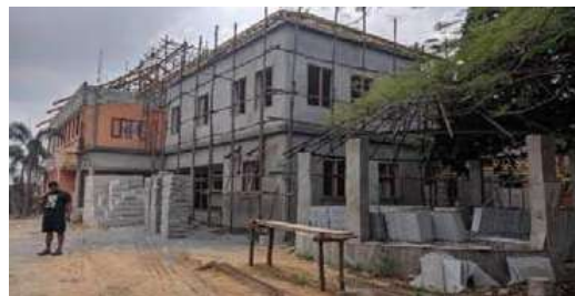
Fig. 8. New construction of sankalp school.
