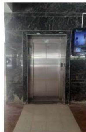
Fig 8. Lift entry with minimum level difference
