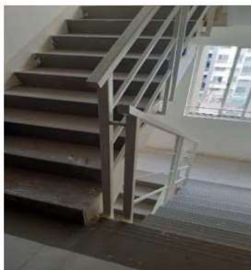
Fig 6 - Staircase with continuous railing
